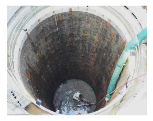
Figure 13 Example of shaft excavation in ECBF (Project Hobson)
