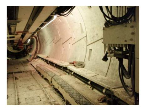
Figure 2 Typical lining using pre-cast gasketed segments (Rosedale Project)
