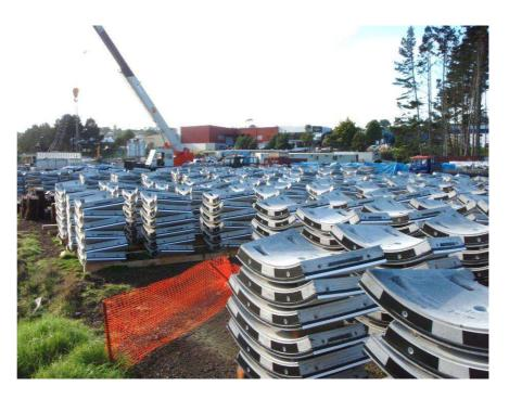
Figure 3 Tunnel segments being stored ready for use at the Rosedale Project construction shaft.
