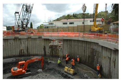
Figure 15 Construction of the shaft walls for Project Hobson pump station.
