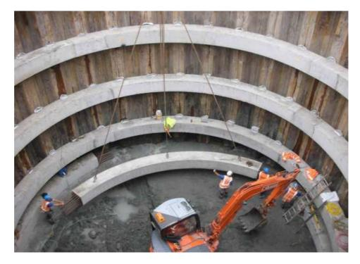
Figure 12 Typical circular construction shaft in soft ground before excavating down into underlying East Coast Bays Formation rock (Rosedale Project)
