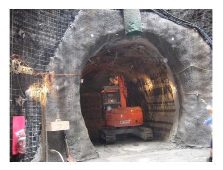
Figure 7 Typical excavation methods for the de-aeration tunnels. Installation of rock bolts and shotcrete lining are visible (Project Hobson)
