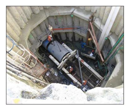
Figure 5 Set up of pipejacking launch shaft for SW Interceptor
